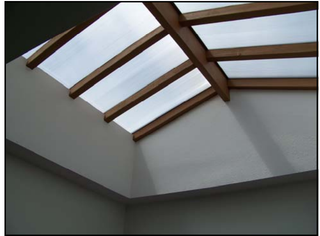
Skylight Above Stairway
