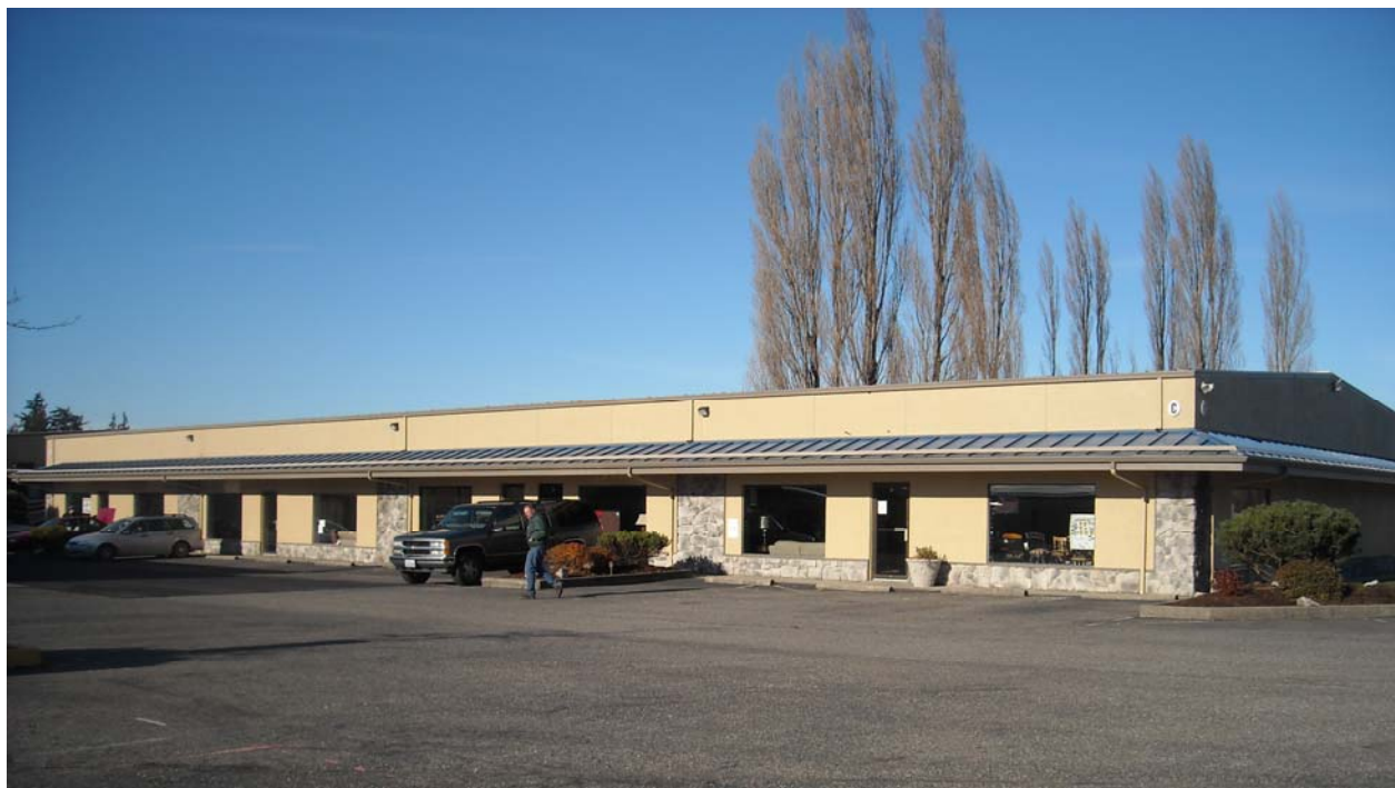
Building C: Office, Warehouse and Industrial
